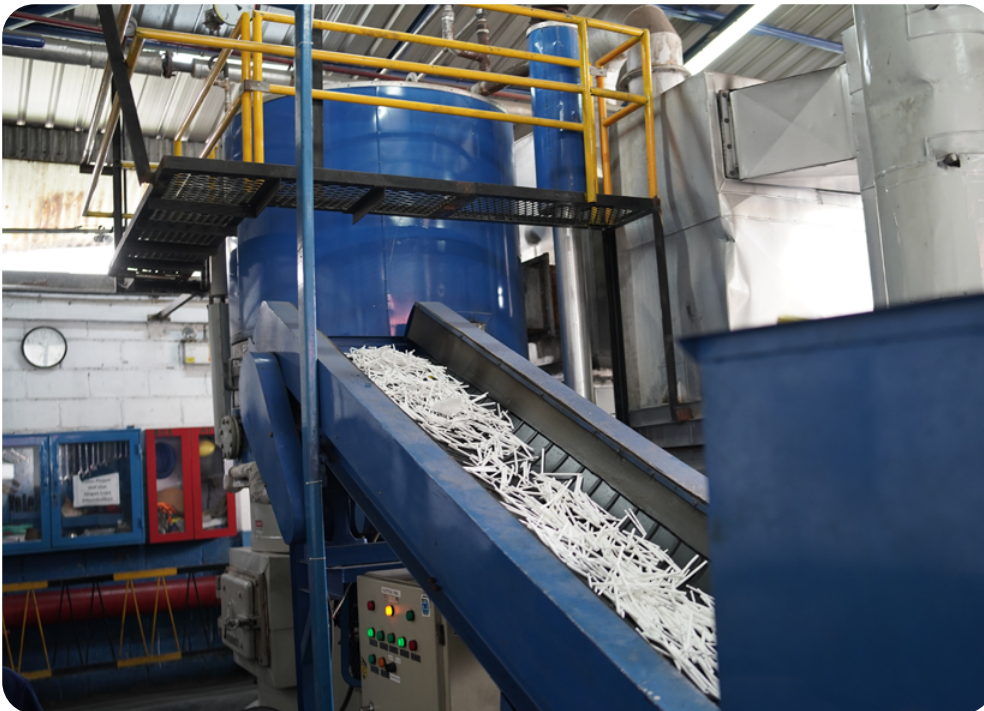
Biomass boiler at Filtrona Indonesia
